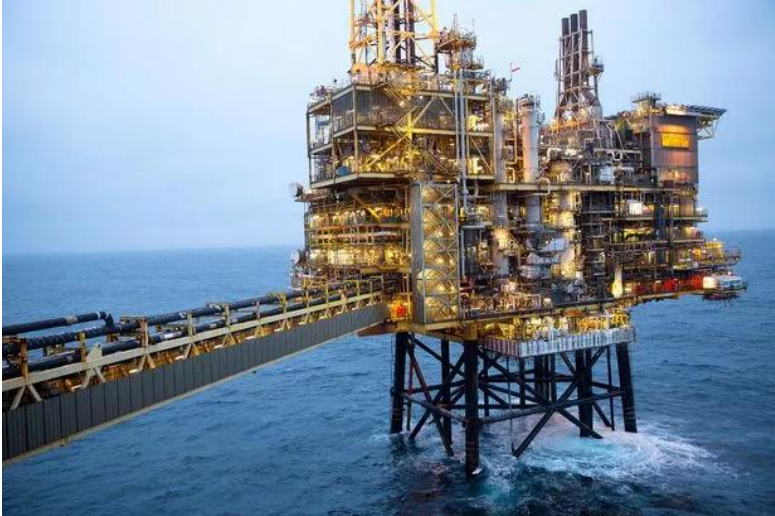
EPCC Brownfield repairs order and modifications across 20+ assets for a variety of customers across the North Sea
