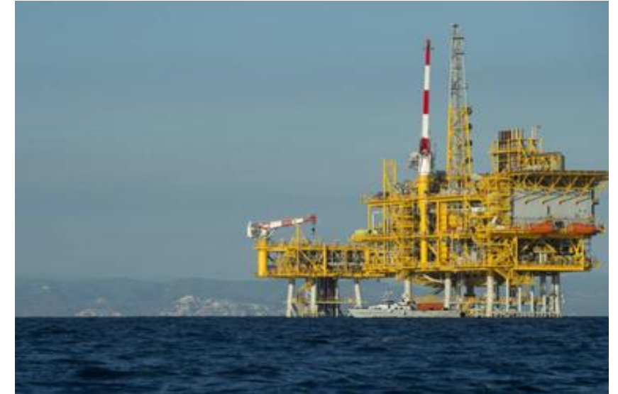
Delivery of Well P&A for 13 platform wells offshore Spain
