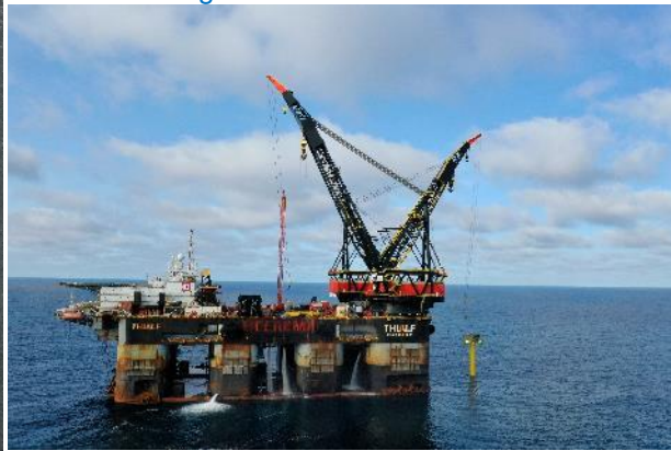
Thialf during B10 platform installation
